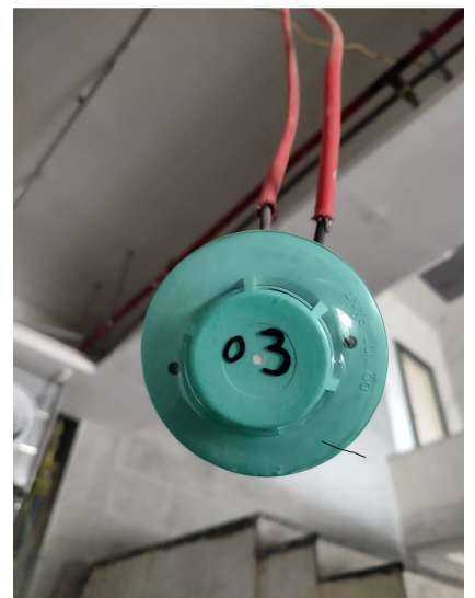
FIRE8325-Fire&Safety -Smoke Detector Addressable -No's
