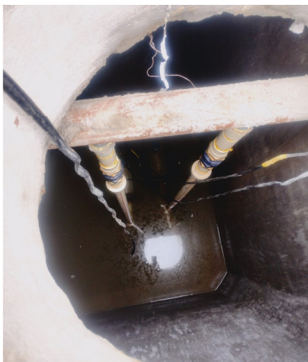
PLUM2237-Plumbing-Dewatering self - Priming mono-block pump-3 phase 3HP-No's
