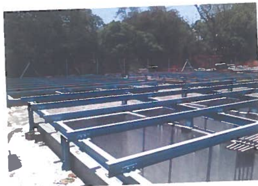
Newly constructed cemented pits
