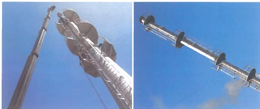
Pictures of chimney erection
