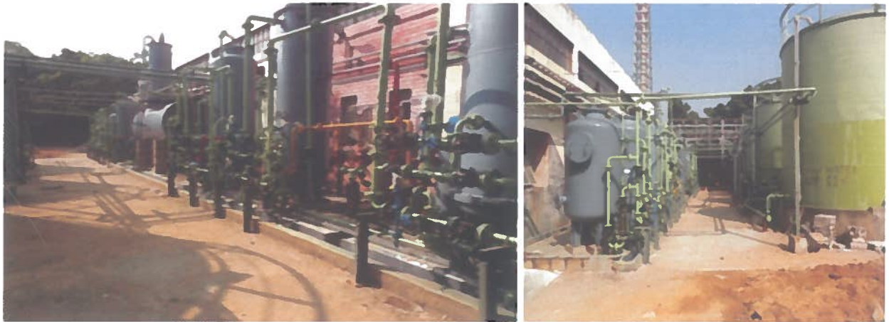
View of the new DM plant
