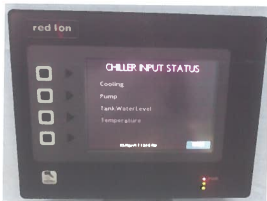
Touch Screen HMI Display provided at Instrument Room Control Circuit Located Inside the Chiller Unit
