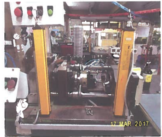
Safety light curtains installed on the End Cap Welding machines.
