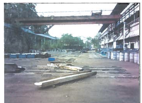
The storage yard after completion of cutting & removing structural
