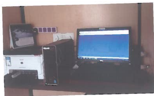
Gas Monitoring System
