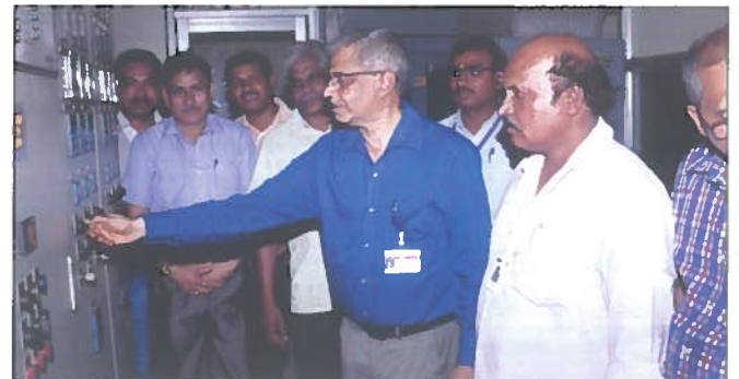
Shri G. Kalyanakrishnan, Chairman & CE, NFC switching on the Board to inaugurate sintering furnace at CFFP-P.
