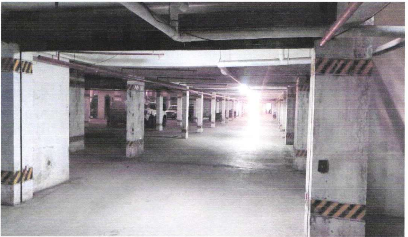
CELLAR FLOOR SPRINKLER SYSTEM INSTALLED
