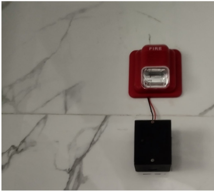
FIRE5585-Fire&Safety-Hooters-Addressable-No
