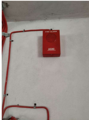
FIRE2644-Fire&Safety-Hooters-Non-Addressable-No's
