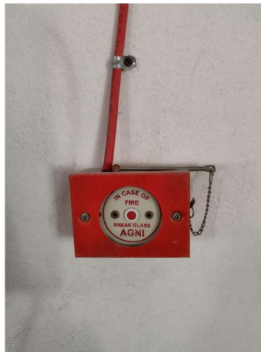
FIRE7360-Fire&Safety-Manual call point-Non-Addressable-No's
