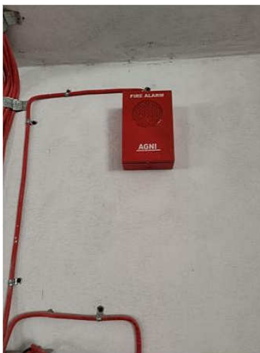
FIRE2644 -Fire & Safety- Hooters - Non Addressable-Nos.
