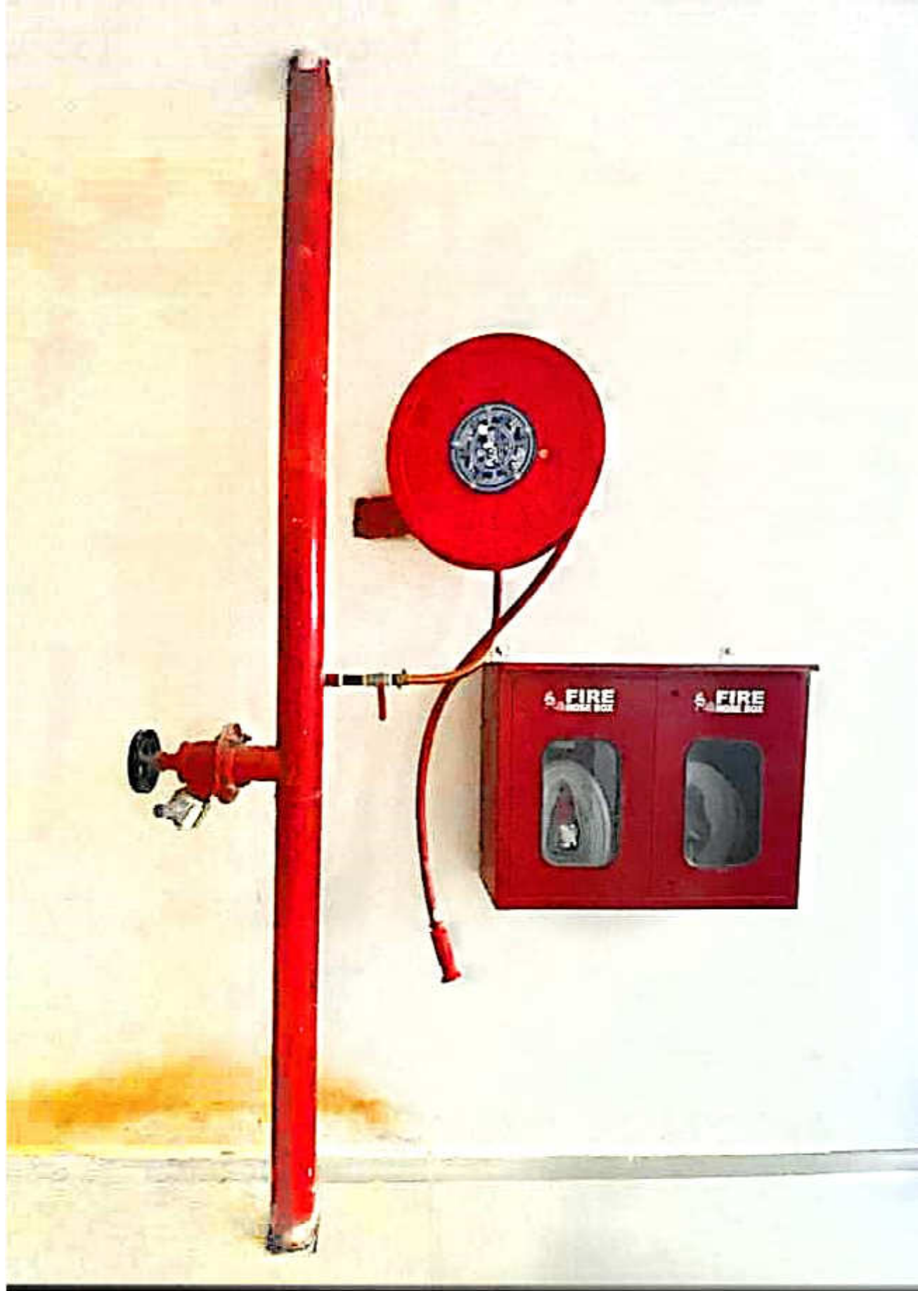
A typical picture showing Downcomer, Hose reel drum & Fire hose box (double door) installed at site.
