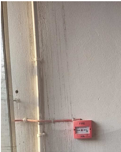
FIRE7360-Fire& Safety -Manual call point -Non addressable-Nos
