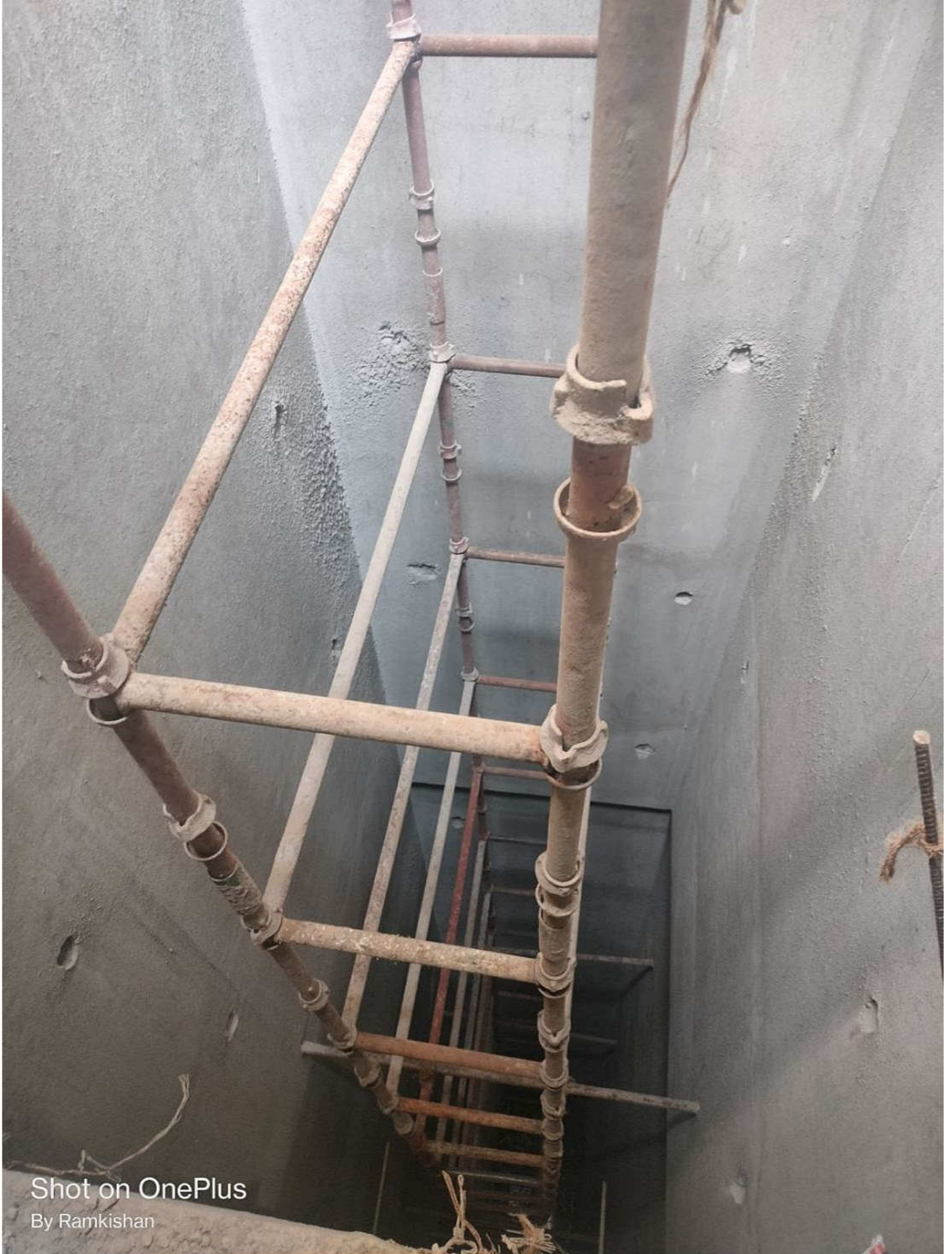
A typical picture showing Cuplock scaffolding erected for Installation of Lift at site.
