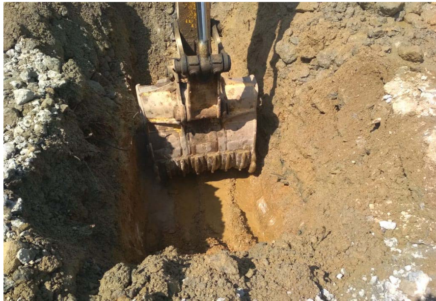
Photograph - 4: Excavated Trial Pit TP-4 Location
