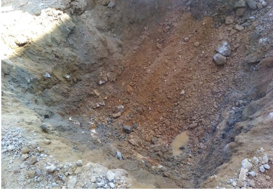
Photograph - 1: Excavated Trial Pit TP-1 Location
