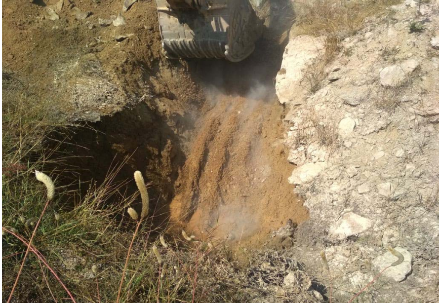
Photograph - 7: Excavated Trial Pit TP-7 Location
