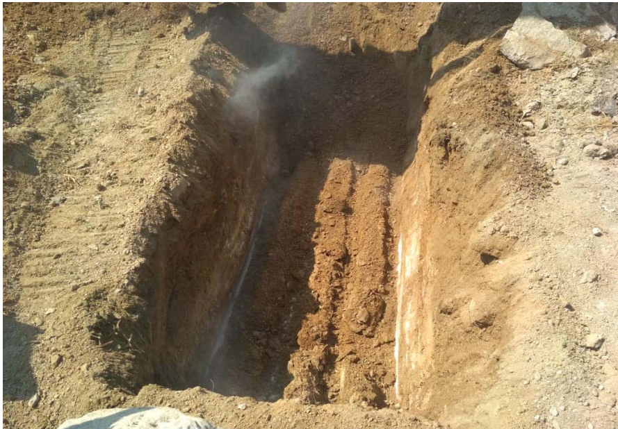
Photograph - 6: Excavated Trial Pit TP-6 Location
