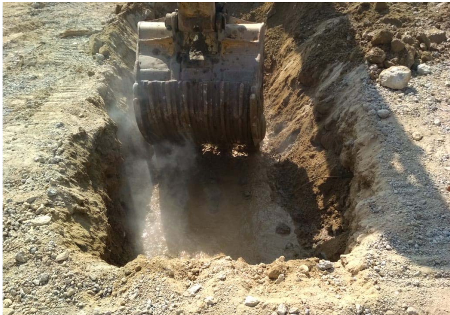
Photograph - 2: Excavated Trial Pit TP-2 Location
