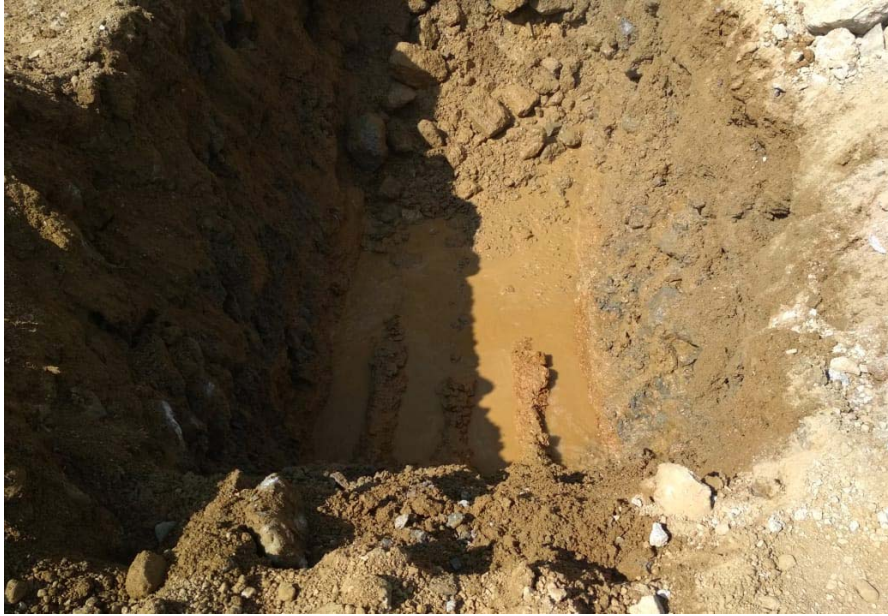
Photograph - 3: Excavated Trial Pit TP-3 Location
