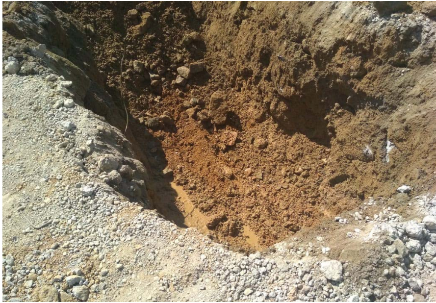
Photograph - 5: Excavated Trial Pit TP-5 Location
