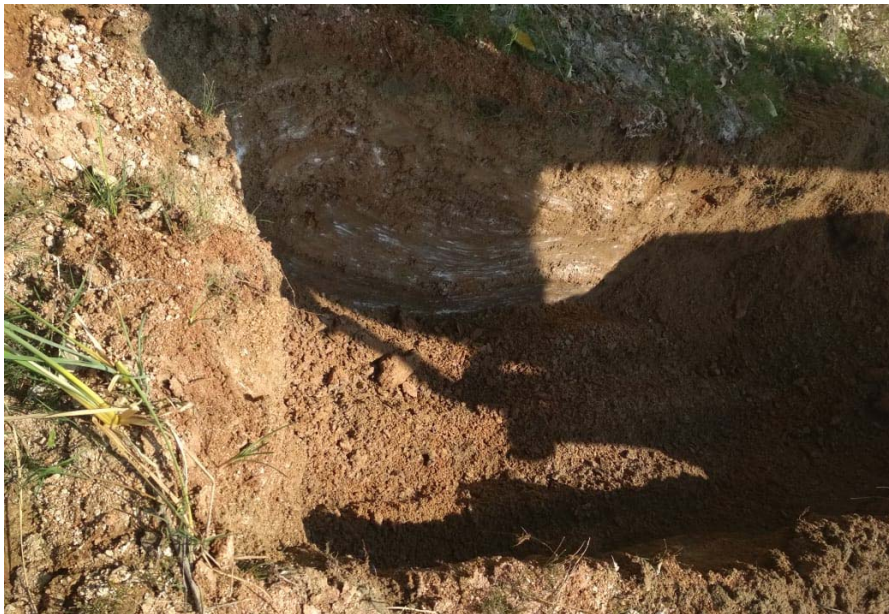
Photograph - 8: Excavated Trial Pit TP-8 Location
