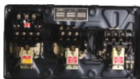
Interior View of MK1 FASD
