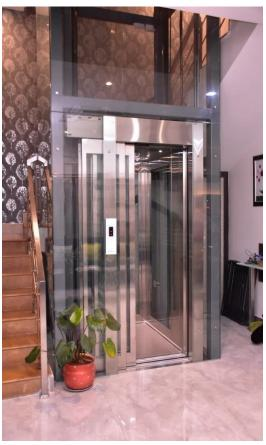
Sub: Supply, Installation, Testing, commissioning and Maintenance of 1No Rosh Vegam Model (MRL Gearless) Lift.
