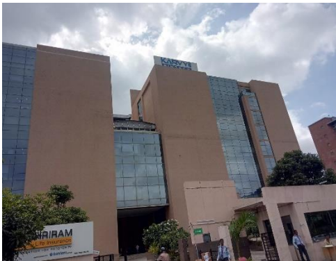
External View of Subject Property
