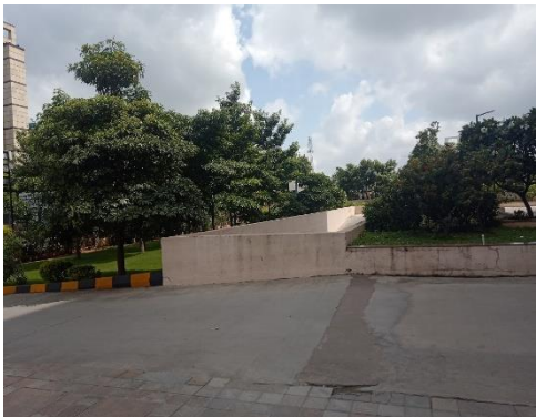
External View of Subject Property
