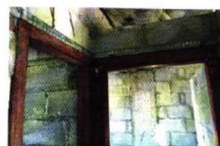
L-shape steel lintel
