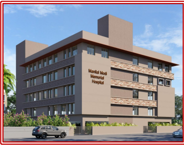
Manilal Modi Memorial Hospital 75 bed, 45,000 sft Hospital building on 1/2 acre, Genome Valley, Hyderabad.
