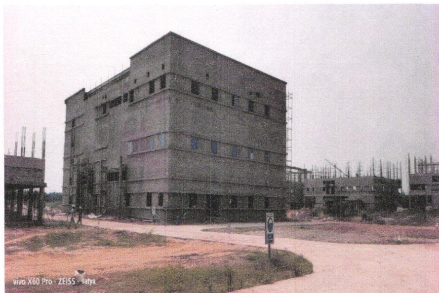
PRODUCTION BUILDING & RAW WATER TANK AT SANVIRA BIO SCIENCES PVT, LTD.
