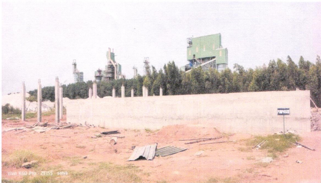
QUARTERS BUILDING AT SIRIUS TRANSPORT PVT, LTD.
