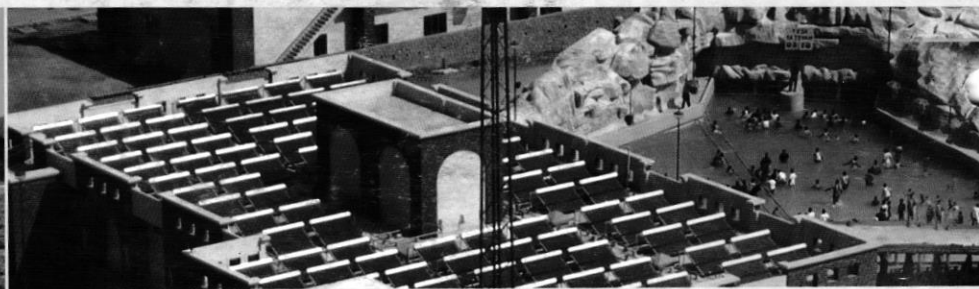
Solar pool heating system (100000 Lpd) installed at Wonderla Amusement Park, Bangalore
