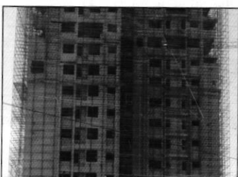
SRR Project Vijayawada
