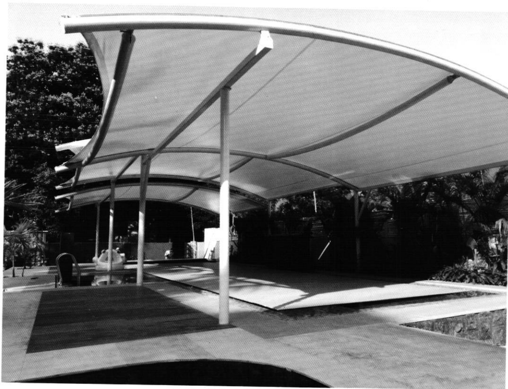
Swimming Pool, Residence
