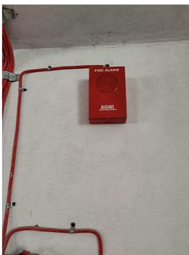
FIRE2644 -Fire & Safety- Hooters - Non Addressable-Nos.
