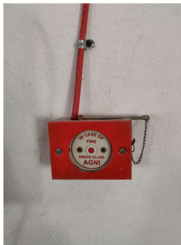
FIRE7360-Fire&Safety-Manual call point-Non-Addressable-No's
