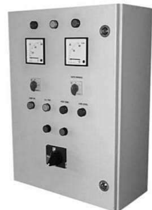
FIRE5063-Fire & Safety-Booster pump panel-12.5Hp-No's
