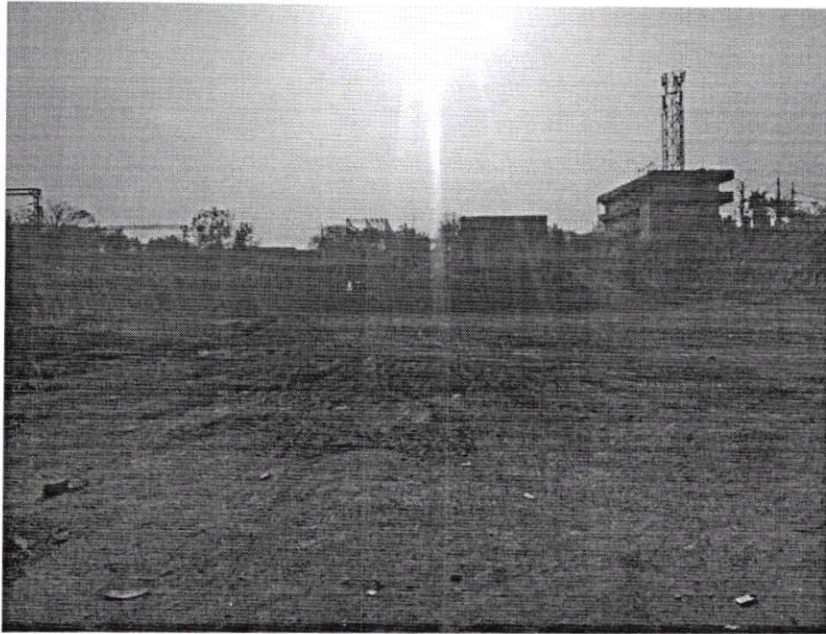
Photograph -1: View of the Site with excavated soil upto 2.0m to 4.0m below the existing ground level
